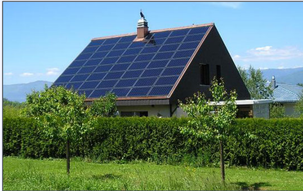
Solar Photovoltaic (PV)
