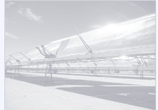
Concentrated Solar Power
