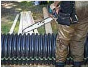
Cutting holes in the pipe
