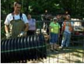
Insert the pipe into the round fence filter.
