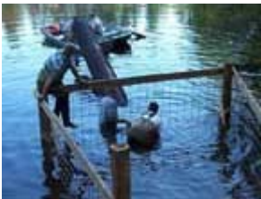
Dropping the round fence into place while securing the pipe in place at the receiver fence.
